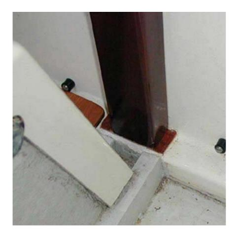
In this case the moulding was very badly damaged, having broken away under the post.
